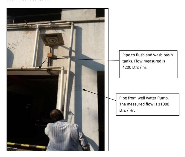
We did not get explanation for balance flow. The flow in pipe on RHS was negligible. The flow through LHS branch could not be measured. Although the metallic valve appears to be closed there must be leakage through this, which needs to be checked.
